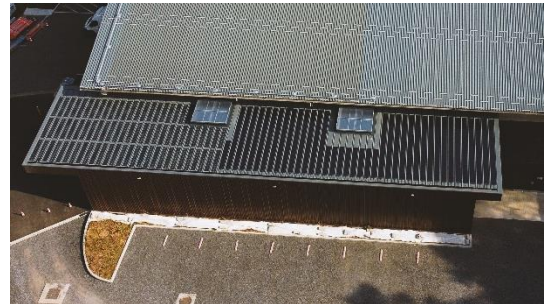
FIGURE 5 : AERIAL PICTURE VIEW OF CRM2 FIELD TEST.
