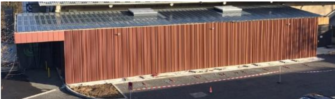
FIGURE 6 : PICTURE OF CRM2 EXTENSION BUILDING, WITH SOLAR PANELS ON ITS ROOF.
